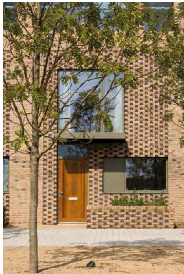
Textured brickwork provides composition and articulation to homes at Abode Great Kneighton
